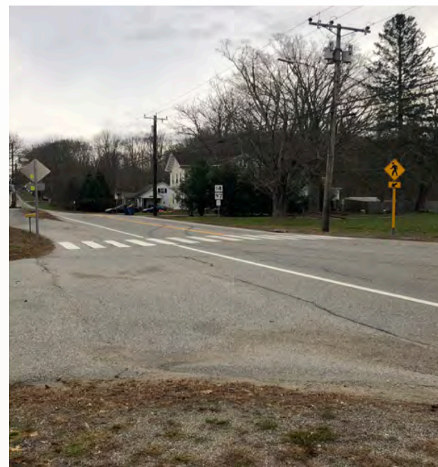
Pedestrian crossing at CT-14/CT-97 (Huntington Road/Palmer Road)
