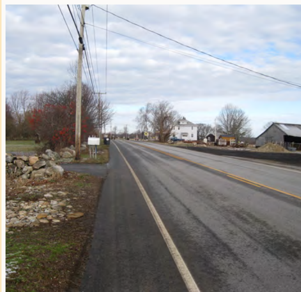
CT-49 south of Hell Hollow Road
