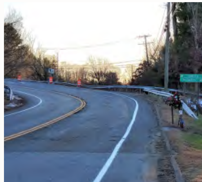
CT-198 (Phoenixville Road) approach to US-6 (Willimantic Road/Hampton Road)
