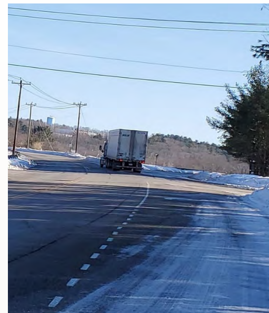
Putnam Kennedy Drive, Technology Park Drive and I-395 sb off-ramp looking south
