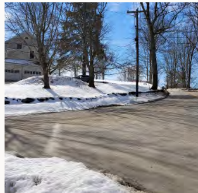
CT-169 (Pomfret Street) at Harrisville Road looking south
