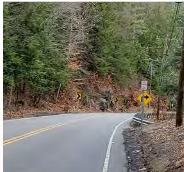
CT-171 (west of Bigelow Brook Road)- Looking east
