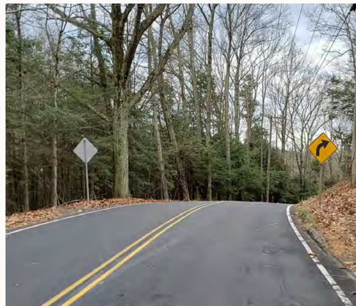
CT-197 (west of Woodstock Town line)- Looking east
